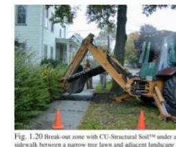
Fig. 1.20 break-out zone with CU-Structural Soil™ under a sidewalk between a narrow tree lawn and adjacent landscape area
